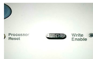
Access Level 3 – The Slide Switch is to the Right
